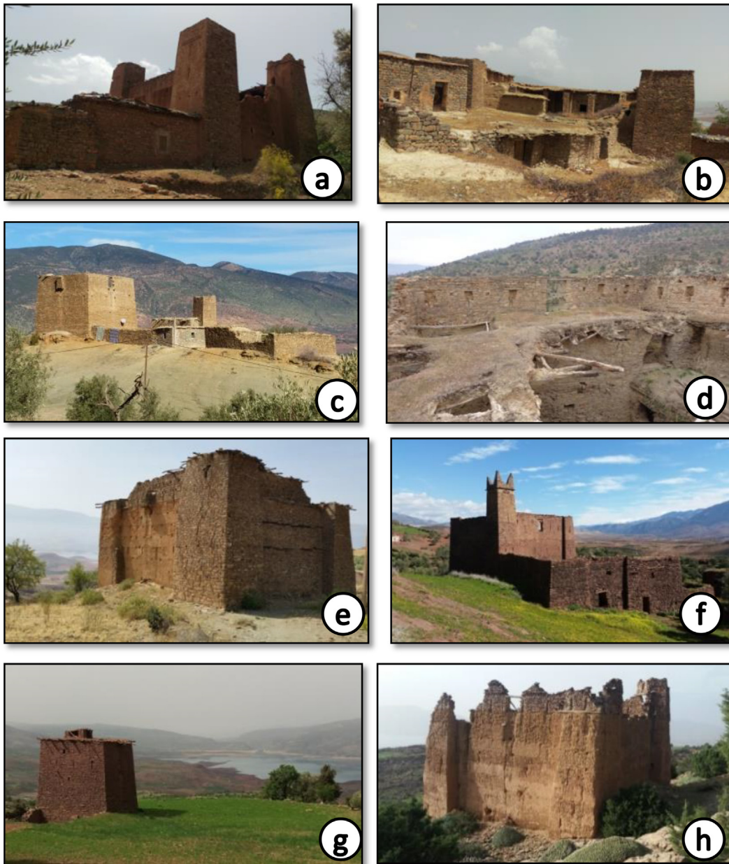
Fig. 12. Granary (Tighremt) of Douar Ait El Bakour with these 4 towers (a), Stone construction associated with the granary of Ait El Bakour (b), Granary of Ait Idir (c), the roof Granary of Ait Idir (d), Granary and Cayda of Ait Halouane (e) (f); Granaries of Ait Mazigh (g) (h).
